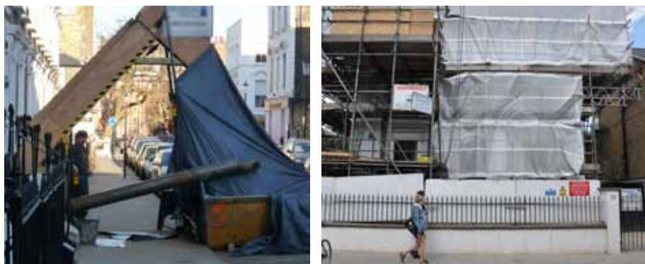
Photographs of good and poor construction site management
